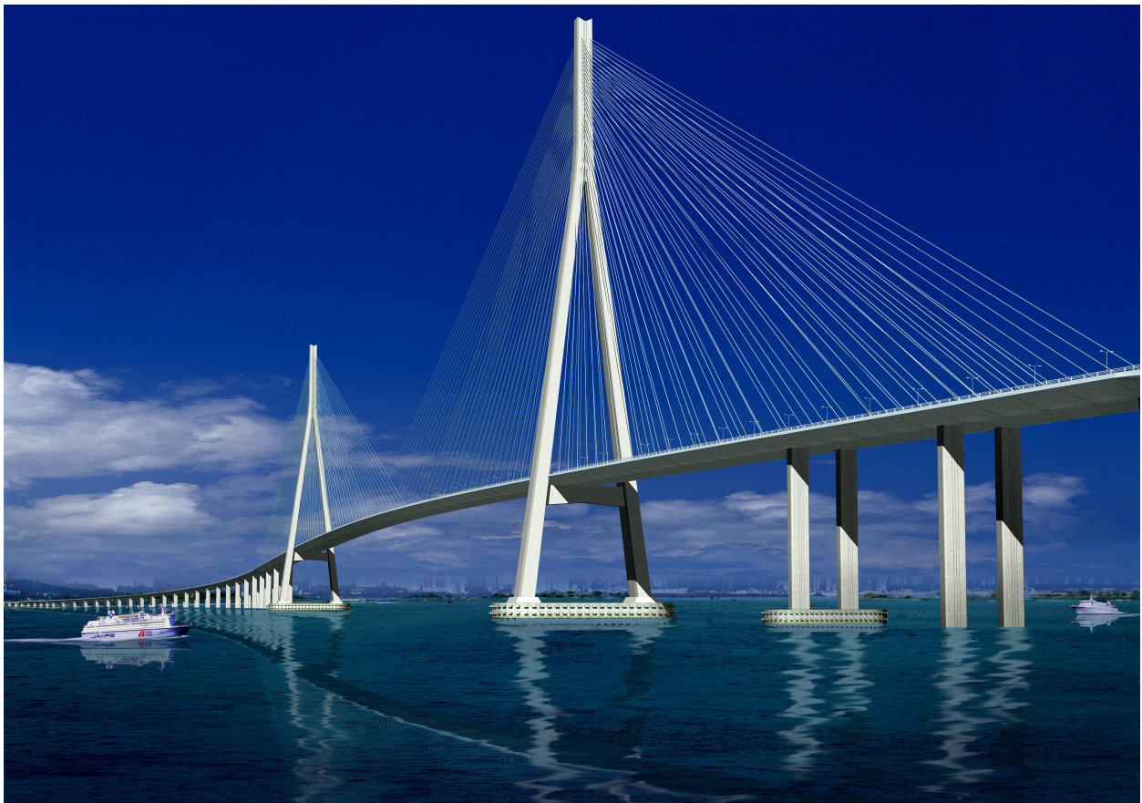
Figure 10: New RM2006 erection control module will be used for Sutong bridge
